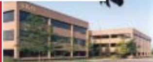
THE GATEWAY BUILDING
