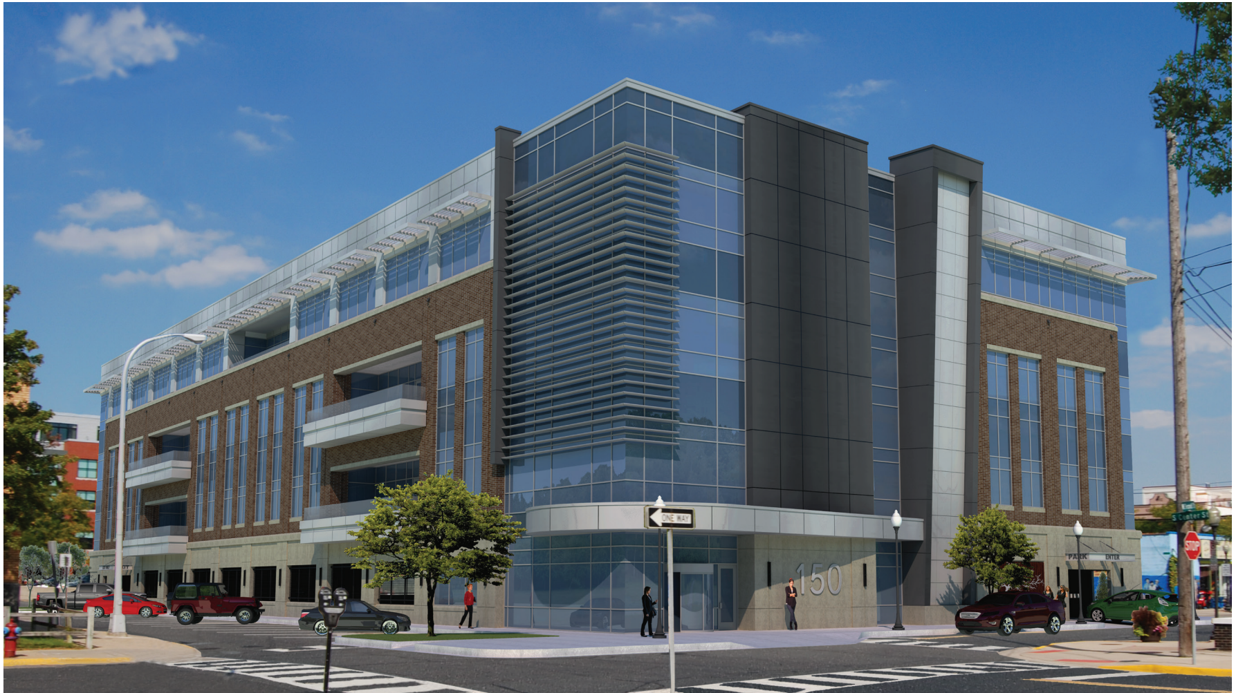
Construction has begun on a 73,920 SF luxury office center at 150 W. 2nd St. in downtown Royal Oak, MI. The developer, Etkin was established in 1982 and has been involved in 9.5 million square feet of high-quality commercial properties nationwide.
